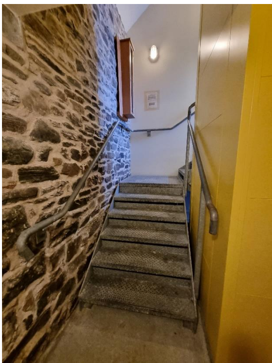
First part of stairs to mini landing
