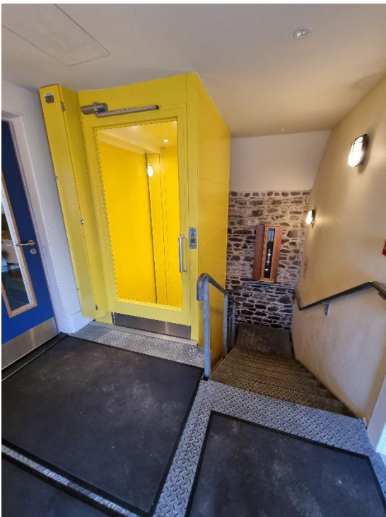
Landing at top of stairs and lift
