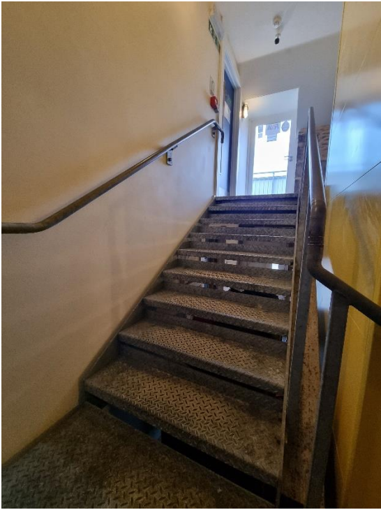
Second part of stairs from mini landing to first floor
