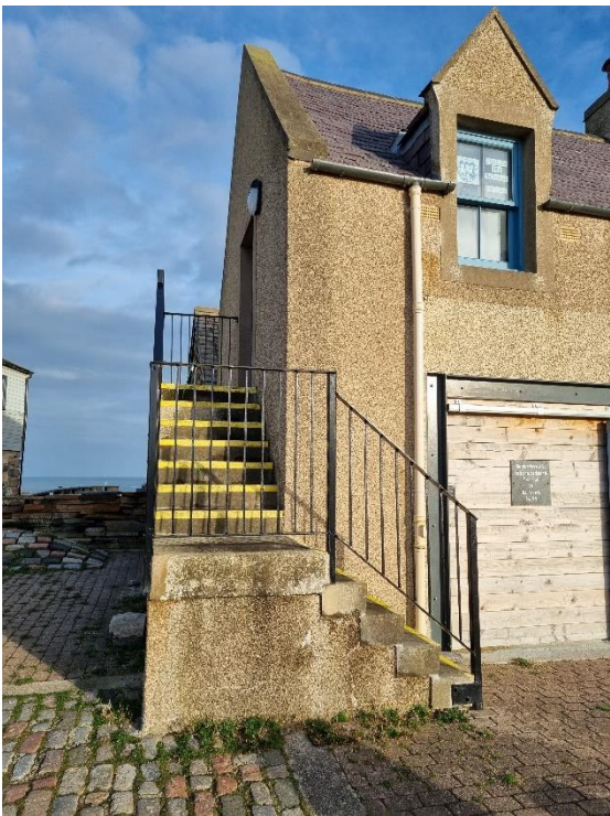
Full staircase leading up to meeting room
