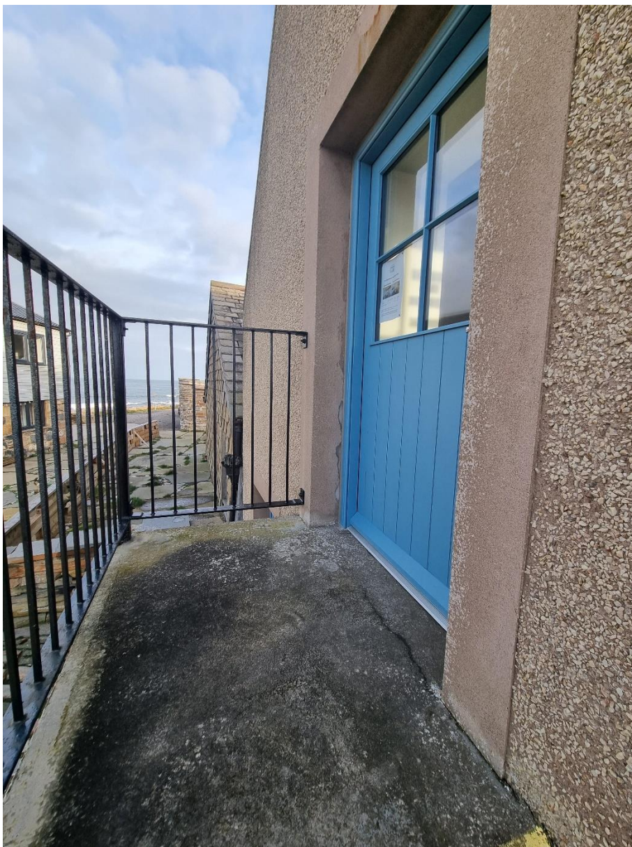
Top of stairs leading to harbour building room
