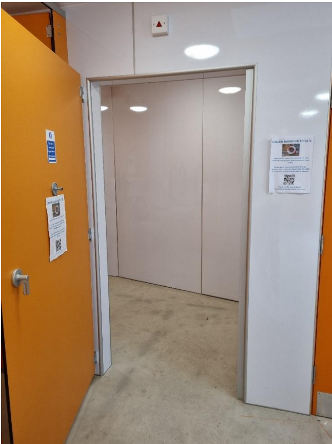
Entrance to Disabled Toilet – Cullen Harbour Toilets
